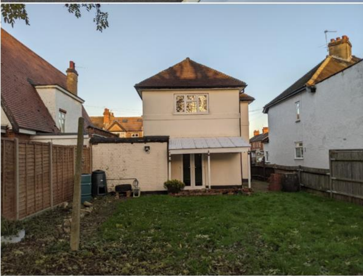
Rear of host site
