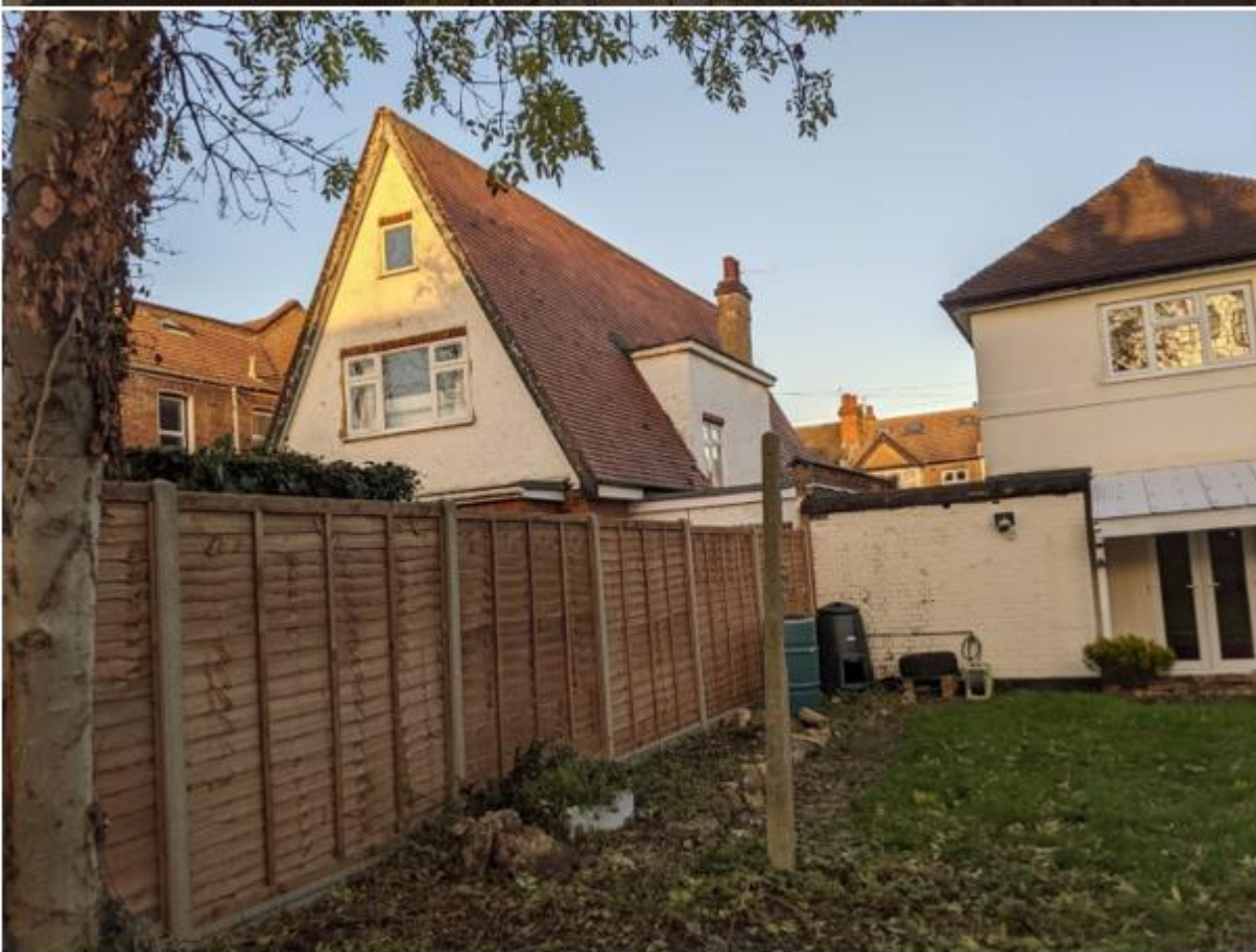
Rear of the site view of no.18
